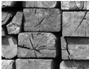
Figure 2 Creosote-treated lumber is found frequently in railroad ties and marine structures
