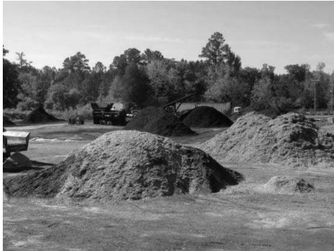
Low permeability pad – strategically sloped to direct water and reduce ponding (with or without runoff collection and treatment).
