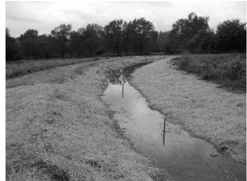
Bioswales / biofiltration structures; stormwater ditches lined in vegetation, cleaned regularly
