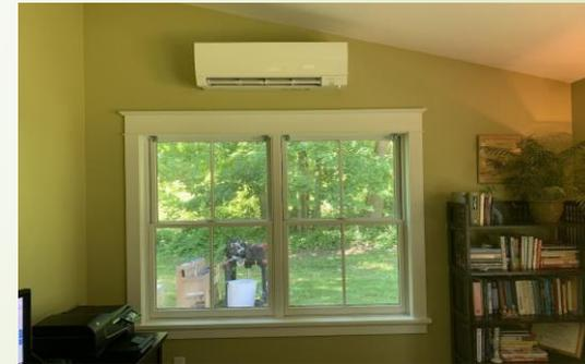
*Photos: Air source heat pump at Sun Creek office building in Stone Ridge*
